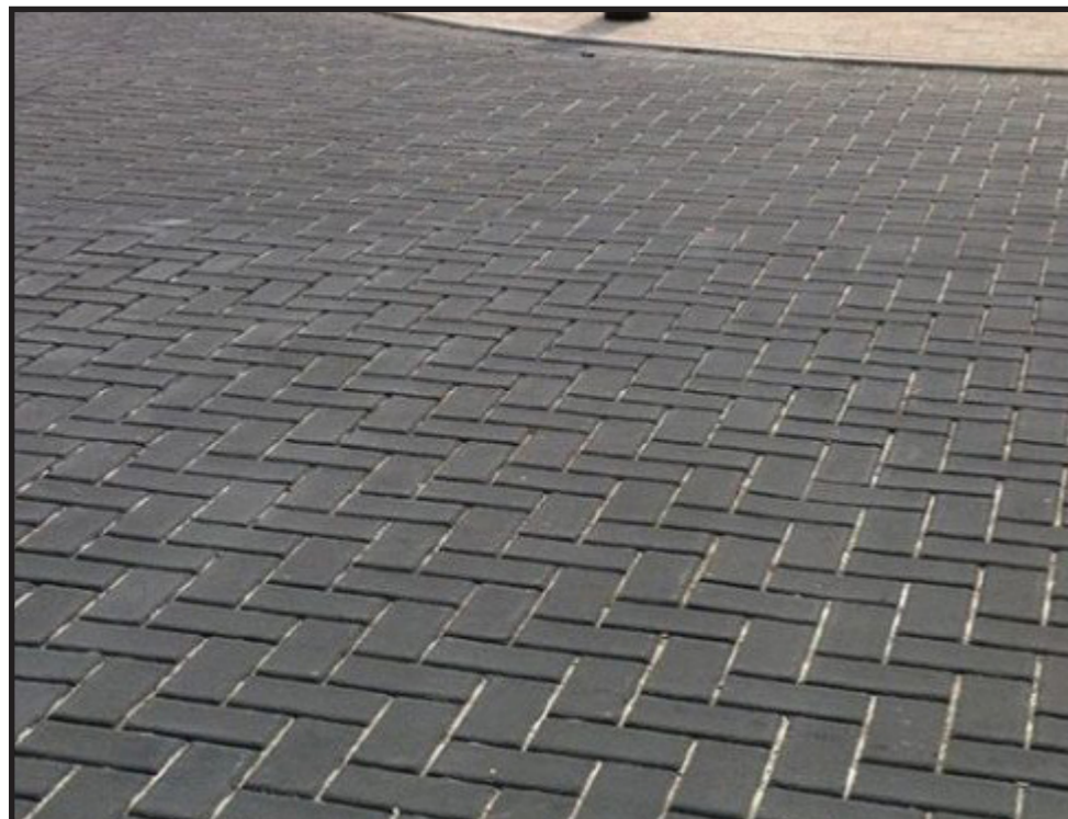
Imprinted asphalt at raised tables at junctions
