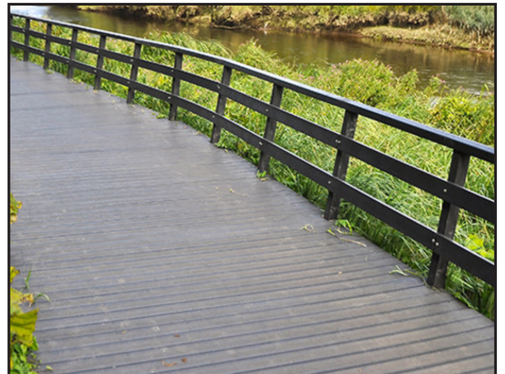
Recycled plastic decking and balustrade to sections of shared footpath/cycleway in the Green Link
