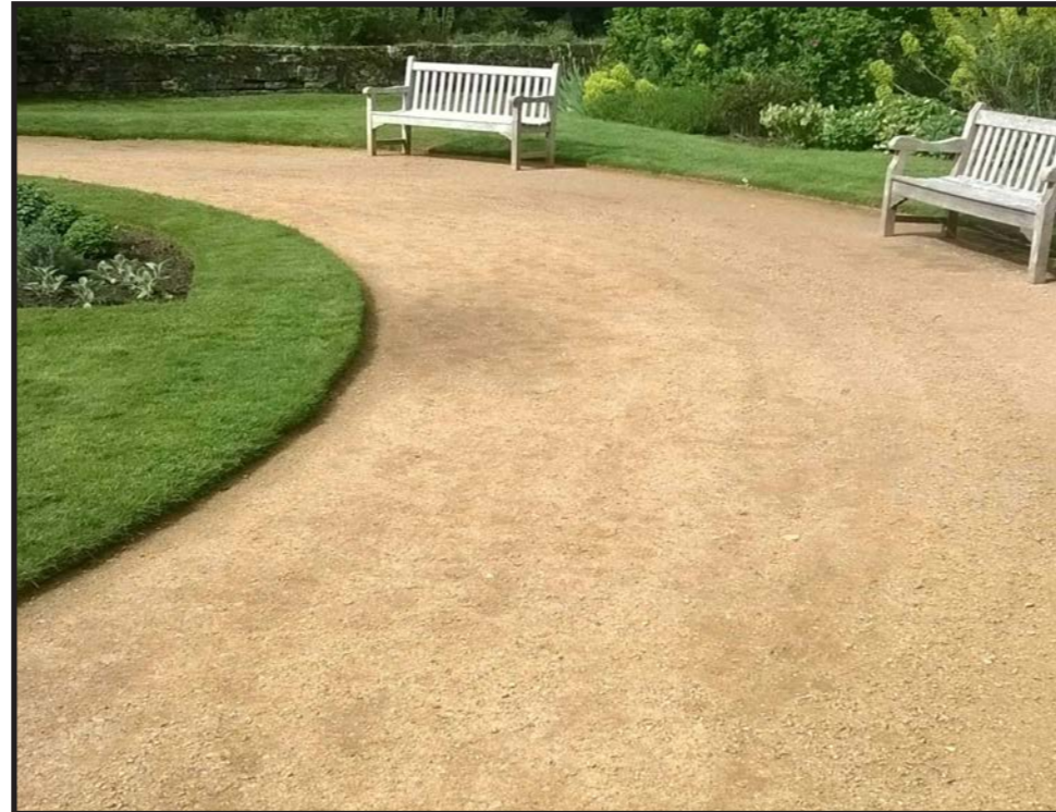
Compacted gravel finish to shared footpath/cycleway within The Village Green.
