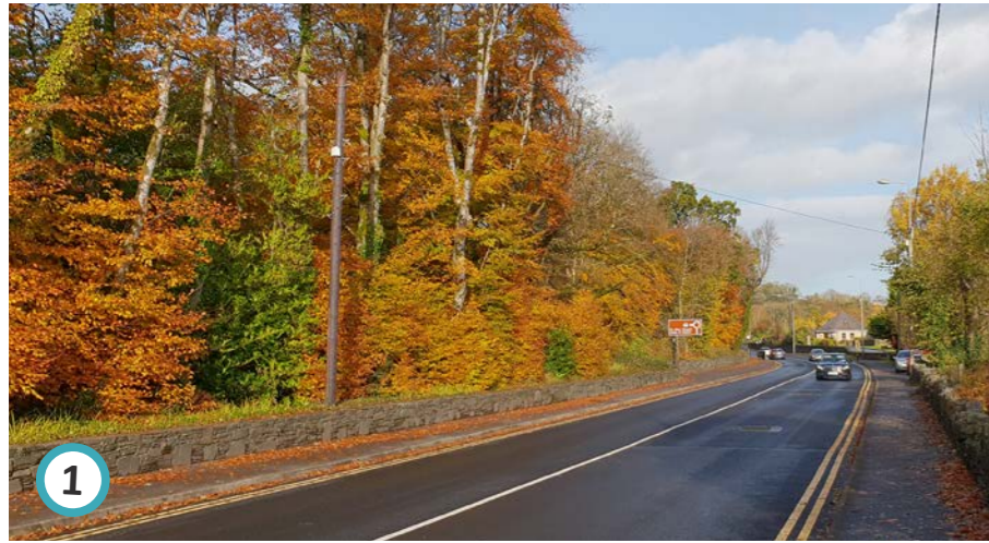
VIEW ON PORT ROAD AND FUTURE ENTRANCE TO THE SITE
