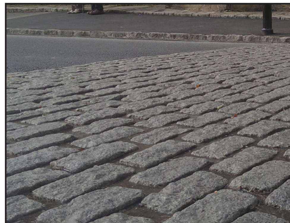
Rumble strips at edges to raised tables at junctions and gateways to shared streets
