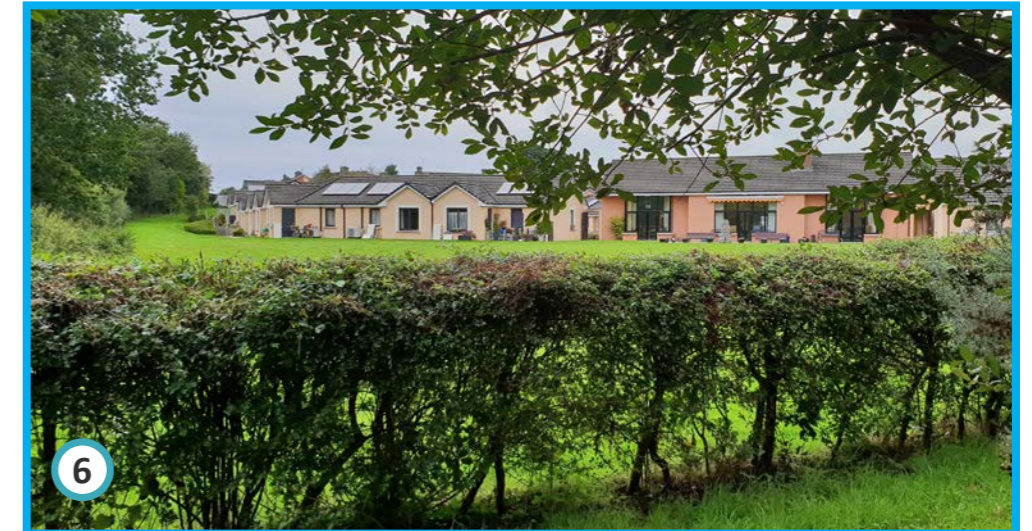
VIEW ON THE NORTH-EAST BOUNDARY- TOWARDS HOLLY CROSS DAY CARE CENTRE
